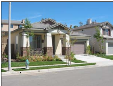
New Housing in Olinda Ranch
